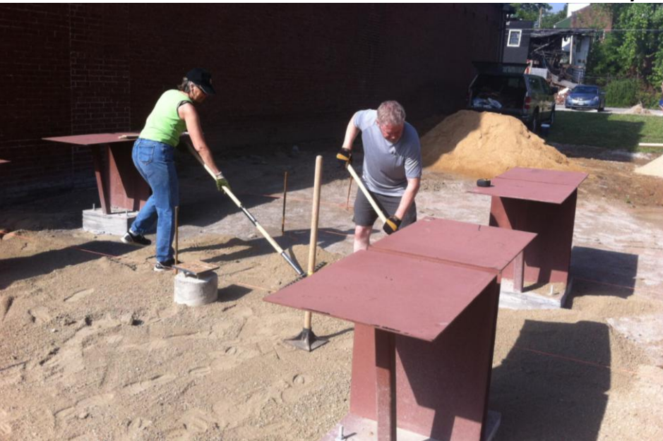
Chess Pocket Park under construction in May
